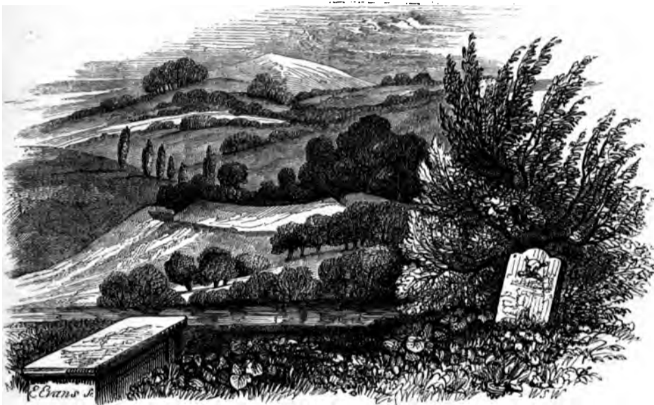
SITE OF THE CASTLE OF THE GOURNAYS AT INLISHCOMBE.
